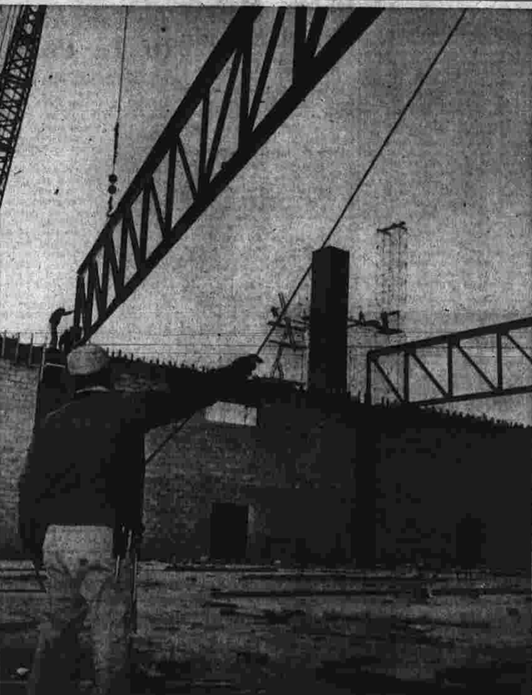
Roof Trusses Placed at New Gym
